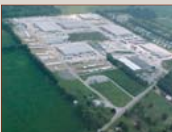
Our 58 acre complex in Warsaw, Indiana
